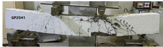
Fig. 14. Cracks at the failure of the GP25H1 beam.
