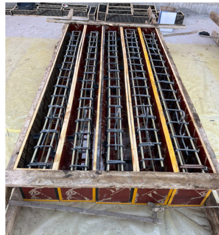
Fig. 4. Wooden molds and steel reinforcement cage of beams.
