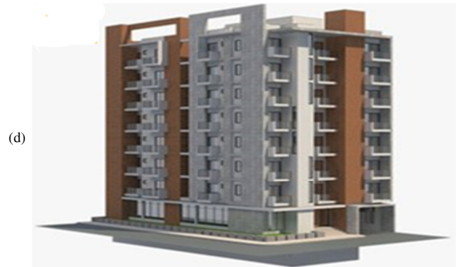
Fig. 2. Selected multi-story case studies: (a) Al-Maaref resident building, (b) Kanan health department, (c) Civil engineering department, (d) Al-Shefaa health department.
