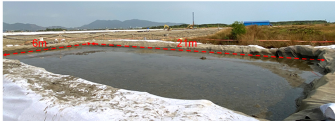
Fig. 3. Preparation of mud pond.
