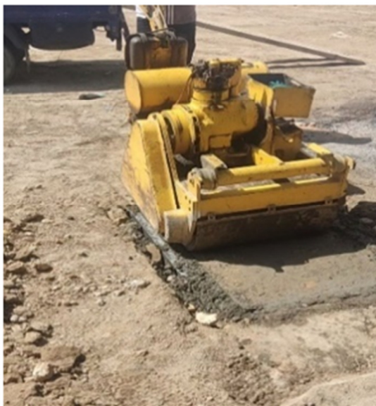
Fig. 3. Compaction of field slab with (BOMAG65).
