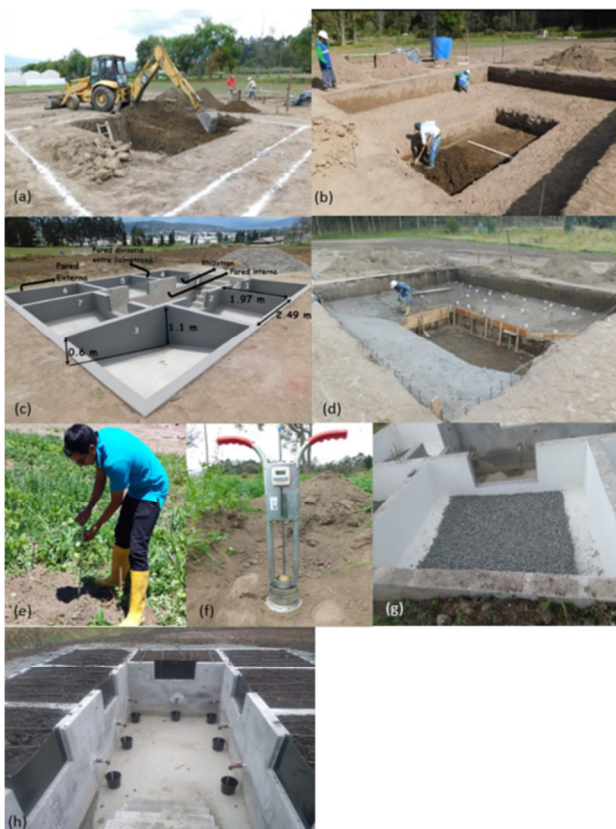
Fig. 3. Construction and calibration of the block of 7 drainage lysimeters.
