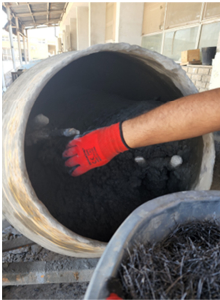
Fig. 7. Steel fiber concrete mix.
