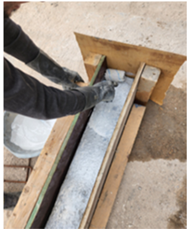
Fig. 4. Applying the adhesive to the old concrete.
