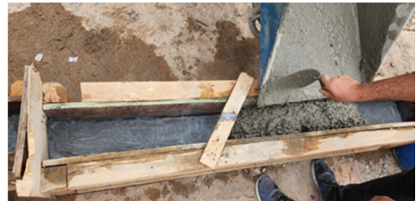
Fig. 5. Pouring the new concrete layer.
