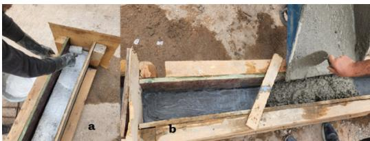
Fig. 3. Producing composite beam (a- Apply the adhesive to the old concrete, and b- Pouring the new concrete layer).
