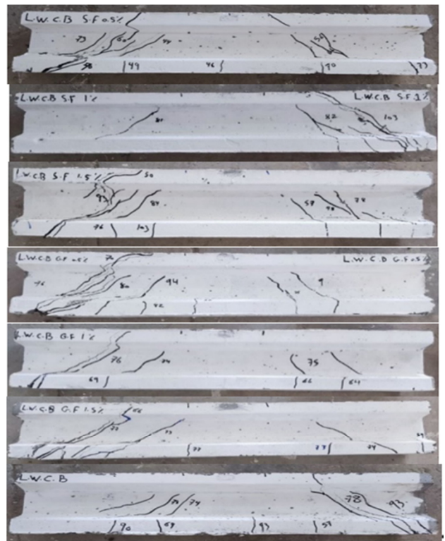
Fig. 12. Crack patterns for lightweight concrete group.
