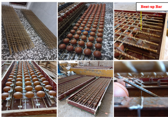
Fig. 3. Picture of the construction of test slabs.
