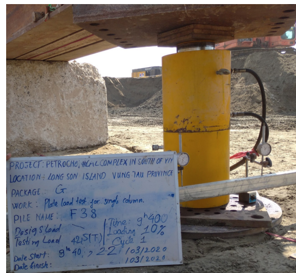
Fig. 5. Single plate load test of the trial stone column.
