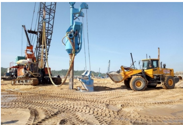
Fig. 3. Dry bottom feed stone column operation at LSP.
