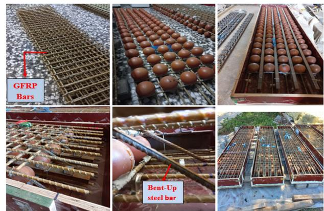
Fig. 3. Pictures of the construction of the test slabs.
