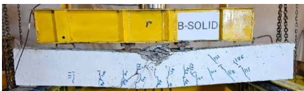
Fig. 11. Mode of failure of B-SOLID beam.
