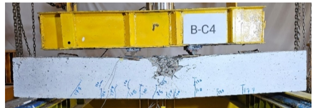
Fig. 15. Mode of failure of B-C4 beam.
