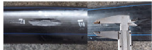
Fig. 4. Pipe with defect (Pipe III).
