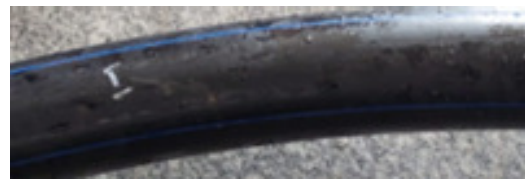
Fig. 2. Crack free pipe (Pipe I).
