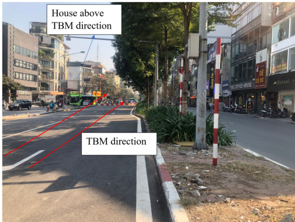
Fig. 1. TBM will pass through the houses above (from Station 9 to Station 10).
