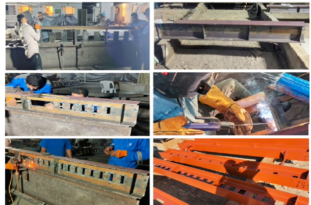
Fig. 6. Fabrication of expanded steel beam web with openings.
