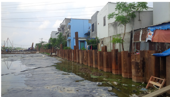
Fig. 2. Construction site with sheet pile protection.
