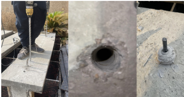
Fig. 3. ETS shear strengthening using CFRP bars.
