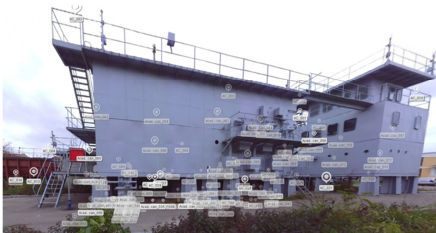
Fig. 4. Example of laser scanning positions.
