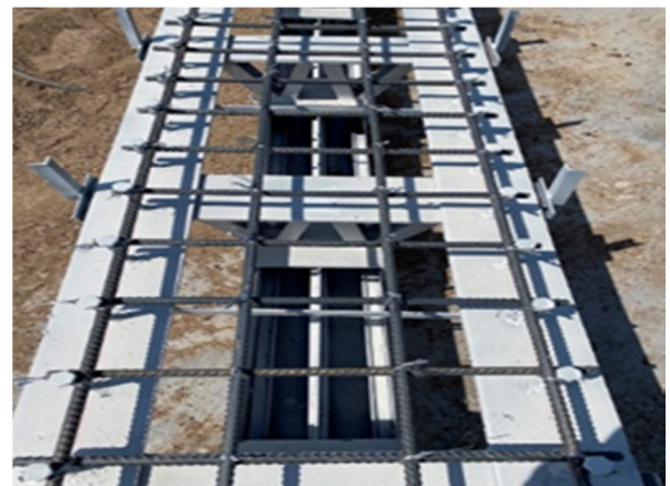
Fig. 3. Main reinforcement of the slab layout.
