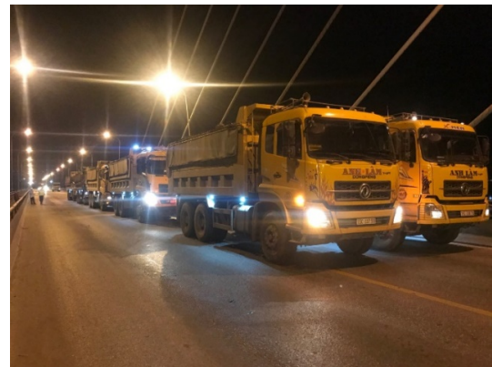
Fig. 2. Static load test to inspection bridge.
