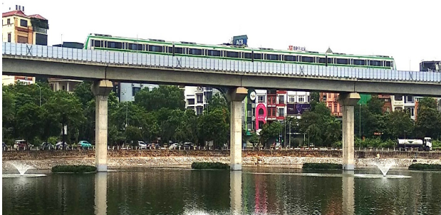
Fig. 5. The Cat Linh-Ha Dong urban railway bridge.
