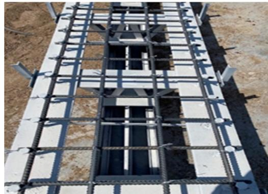
Fig. 3. Main reinforcements of the slab layout.
