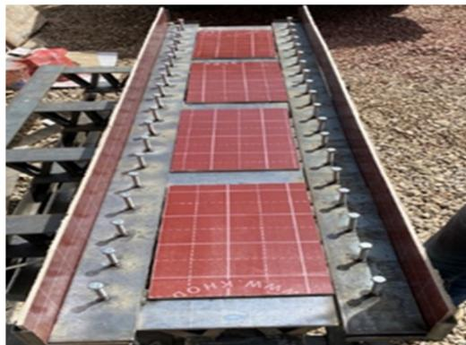
Fig. 2. Stud shear connector distribution.
