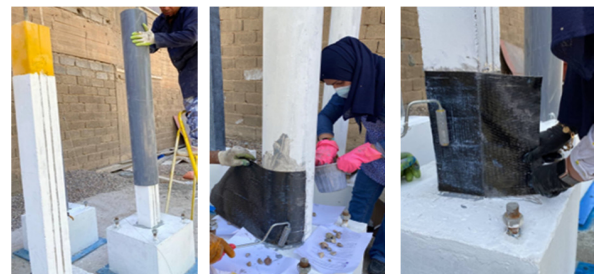
Fig. 7. Circularization and CFRP-EB technique.
