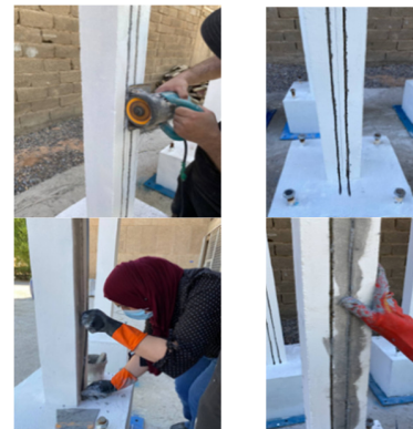
Fig. 6. NSM-CFRP technique procedure.
