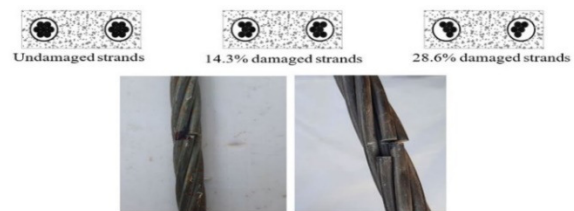
Fig. 1. Patterns of damaged strands in the tested girders.
