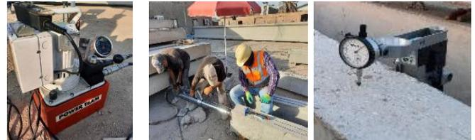
Fig. 3. Post-tensioning process.
