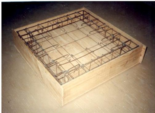
Fig. 1. The Reinforcement cage.
