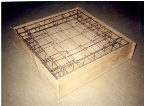
Fig. 1. The Reinforcement cage.
