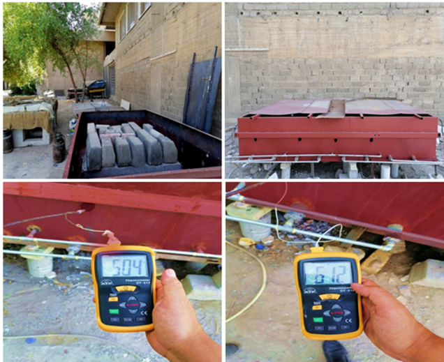
Fig. 3. Furnace and burning procedure.
