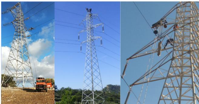
Fig. 10. Maintenance works on double circuit towers with only one of the circuits turned off. Extra care and consideration should be given to the direction of the wind as ropes and pulleys are used to lift tools and equipment to the maintenance spot.
