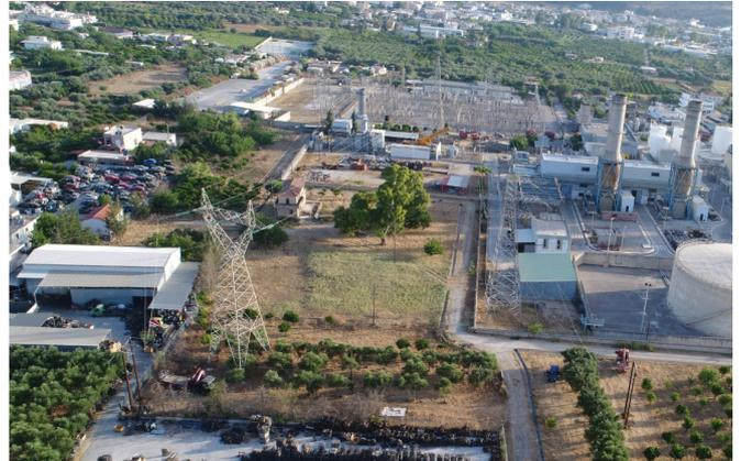
Fig. 22. An overview of the temporary connection of the Vryses-Chania and the Chania-Kasteli circuits using wooden structures, near the Chania Substation and the adjacent power plant.
