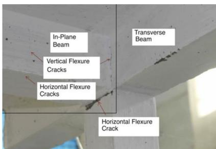
Fig. 22. Vertical and horizontal flexural cracks in in-plane beam.
