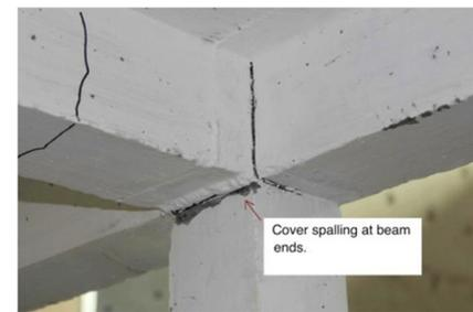
Fig. 25. Spalling of concrete.
