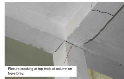
Fig. 24. Flexural cracks at the top end of a column.
