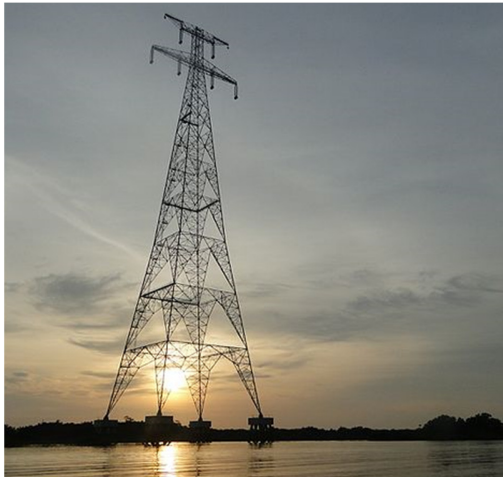
Fig. 1. Tower for large river crossing related to the Tucuruí-Macapá-Manaus interconnection.
