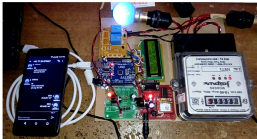
Fig. 5. Hardware implementation of the Android Mobile App-based energy monitoring system
