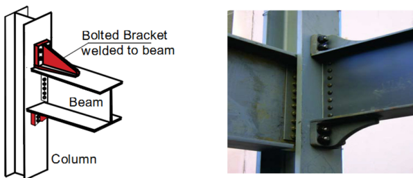
Fig. 5. Bolted bracket and typical connection
