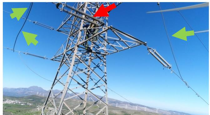
Fig. 5. A direct view of the flashed under insulator (red arrow). Some conductor parts used for phase transposition are also visible (green arrows).
