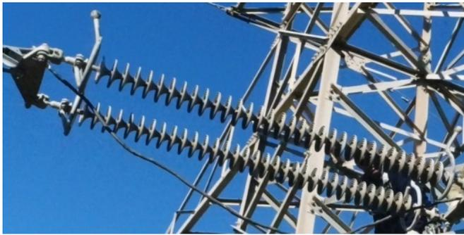
Fig. 8. Even from a small distance, the damage is not visible due to the sheds overshadowing the seath
