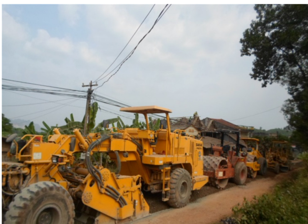
Fig. 2. Picture of on site equipment during the test
