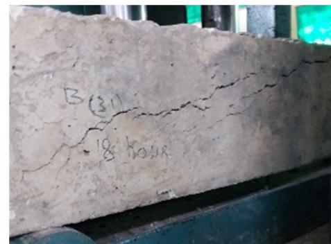
Fig. 13. Cracking in beams
