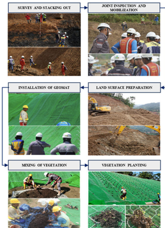
Fig. 3. Implementation of slope protection.
