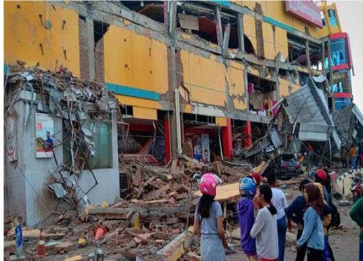
Fig. 1. Collapsed buildings observed after structural failure.
