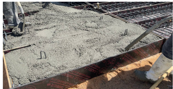
Fig. 4. Installation of reinforcement mesh concrete pouring.
