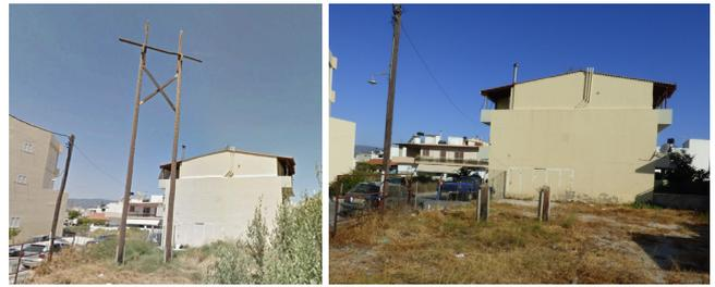
Fig. 3. Removal of an old 66 kV line supported by wooden poles. Left image: the wooden support structure (Screenshot from Google Earth, Image © 2018 Google, © 2019 Google, © 2018 BasarSoft). Right image: the current state.
